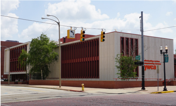
22. Phoenix Building Address: 801 South Saginaw St. Architect: George Pelham, 1966
